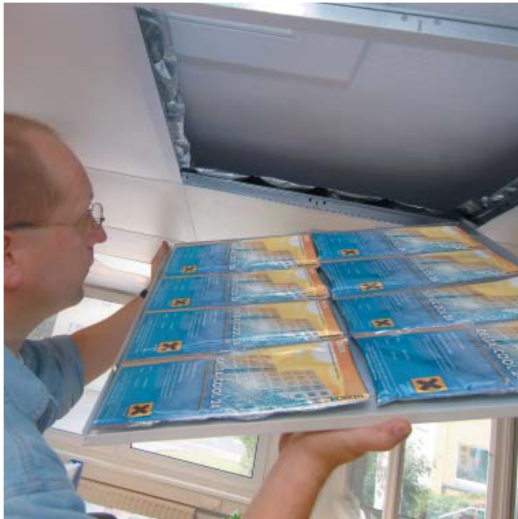
DELTA®-COOL 24 can be easily placed on top of suspended ceilings.
